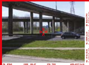
Infrastructure & Road construction
